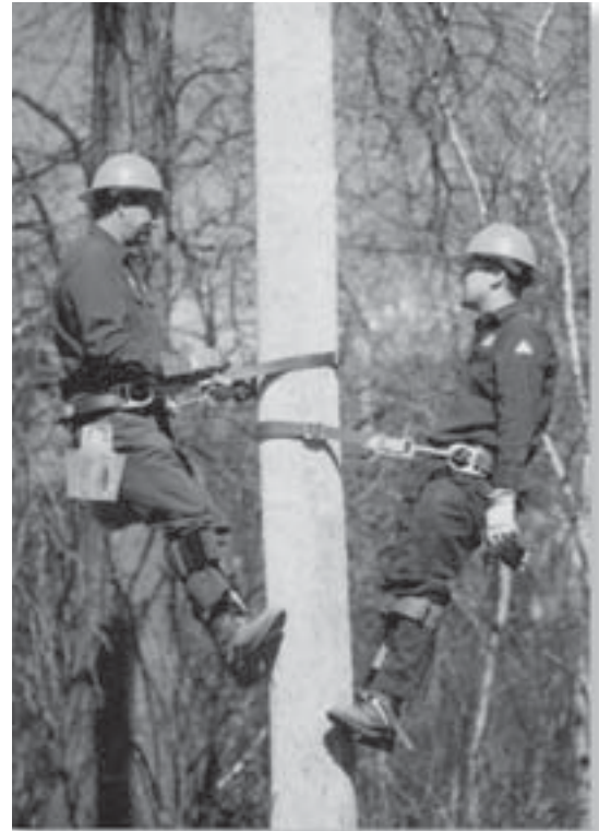
Pole climbing and safety training are regular parts of linemen training at Groton Electric Light, as demonstrated here by Linemen Dave Goodall and Ryan Andrews.
